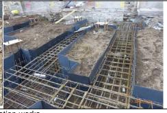
Foundation reinforcement & Shuttering installation works
